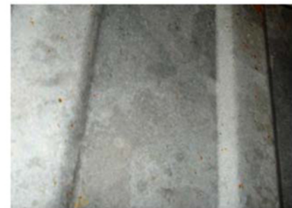
(5.c). The tank walls after washing and cleaning processes with vinegars and gasoline
